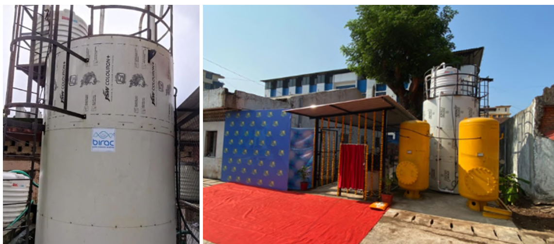
Biodigester using food waste installed at a site in Panaji (Flycatcher technologies, Goa)
